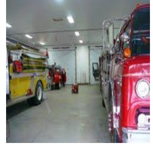
new cement floor in fire hall
