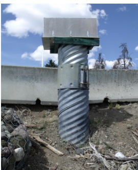
Old Stilling well at culvert
